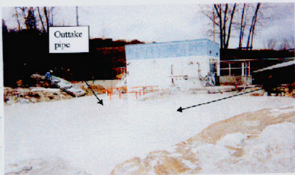
Photo #7: Outtake pipe location at northern end of lagoon #4.
